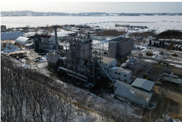
(2nd power plant)
