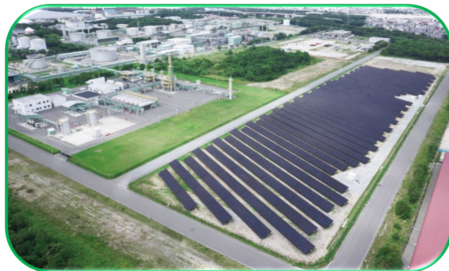
JAPEX Hokkaido District Office's mega-solar power plant site
