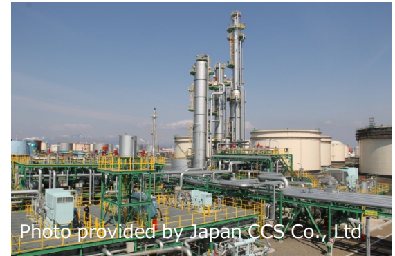
Ground facilities of CCS Demonstration Project at Tomakomai
