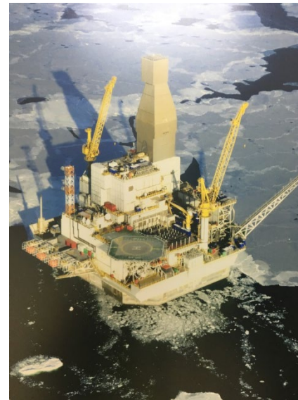
The Arkutun-Dagi Offshore Field Provided by Exxon Neftegas Ltd.
