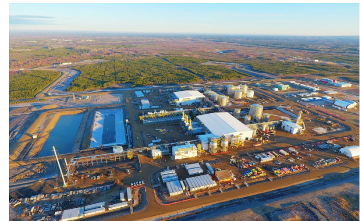
The Central Processing Facility
