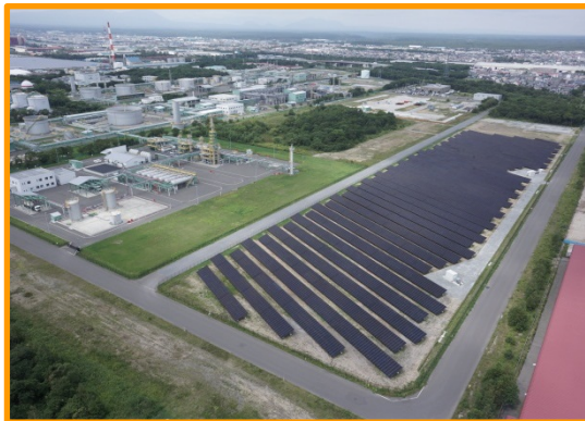
Solar panels at Hokkaido District Office
