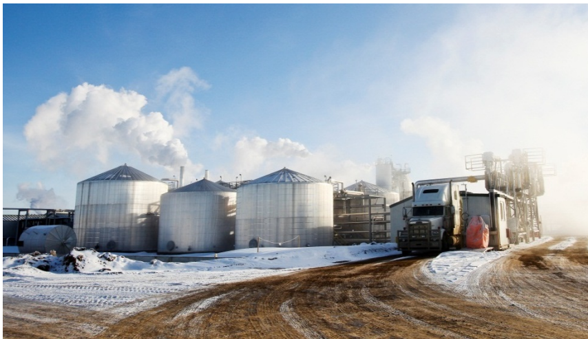
Central processing facility in the Hangingstone Demonstration area
