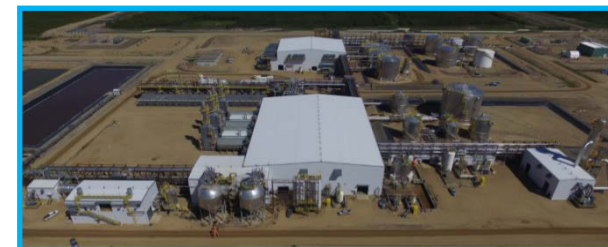
Central processing facility in the Hangingstone Joint Venture area
