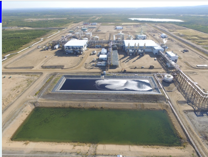
Central processing facility in the Hangingstone Joint Venture area that started production from August 2017
