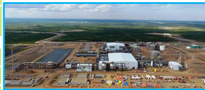
Central Processing Facility for Hangingstone Expansion Project
