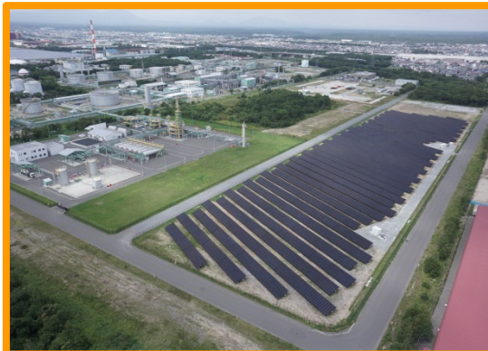
The mega-solar power plant located within Hokkaido District Office site
