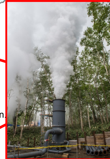
Provisional jet test in Mt. Musa area
