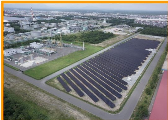
Mega-solar power station at JAPEX Hokkaido district office
