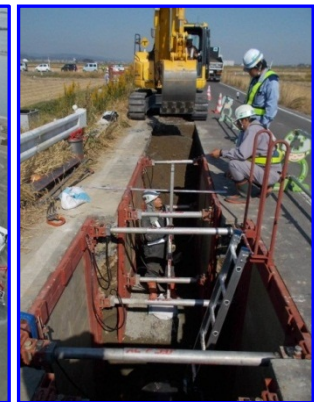
Construction of the connecting pipeline (Oct. 7)
