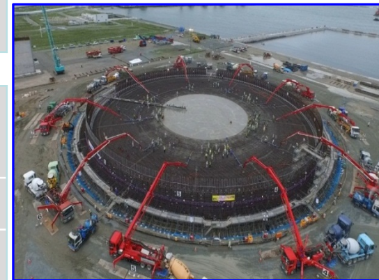
Concrete placement construction work on the Soma LNG tank foundation (June 28-29)
