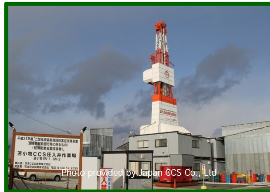
Drilling of CCS observation well
