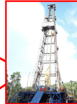
Drilling operation of Musadake area
