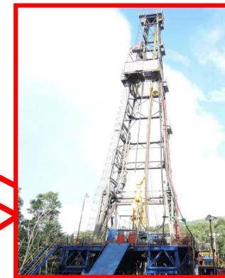
Drilling operation of Musadake area
