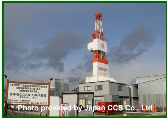
Drilling of CCS observation well
