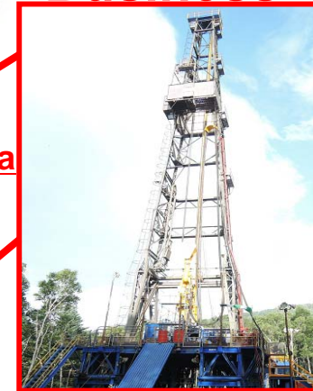
Drilling operation of Musadake area
