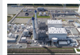
Fukushima Natural Gas Power Plant of the Fukushima Gas Power Co., Ltd.
