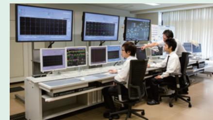
Nagaoka Gas Transmission Monitoring Center
