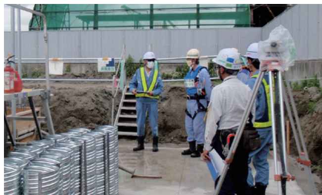
An HSE officer in action at a construction site
