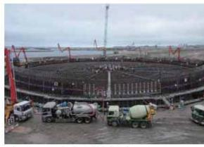
Laying the concrete for the tank's deck slab
