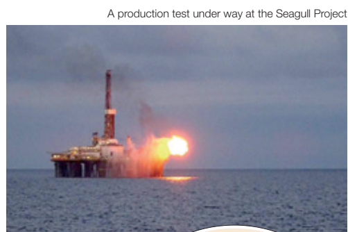
A production test under way at the Seagull Project
