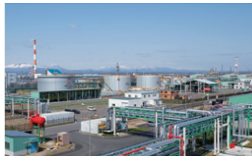
The Yufutsu Plant
