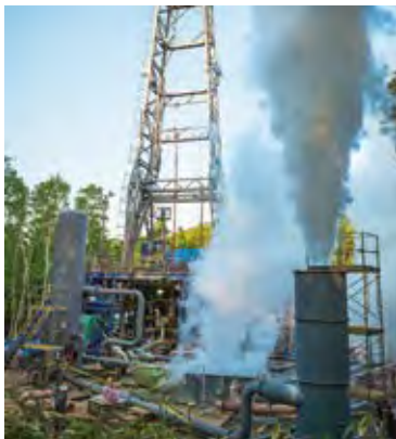
Drilling operation of geothermal exploratory well in June 2015
