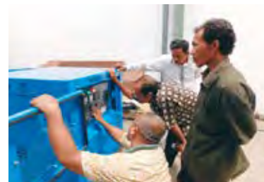
Installing power generation equipment
