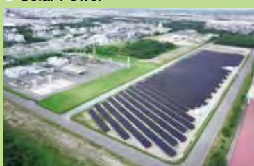
Hokkaido District Office's mega-solar power plant site
