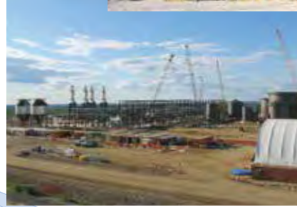
Canada Oil Sands Project
