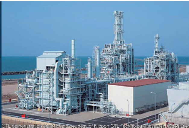
GTL demonstration plant (Photo courtesy of Nippon GTL Technology Research Association)
