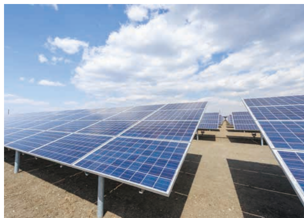
△ Mega-solar power plant in Hokkaido
