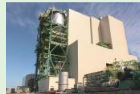
Ozu Biomass Power Plant in Ehime Prefecture
