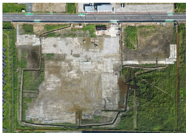
(construction site photo from high level)
