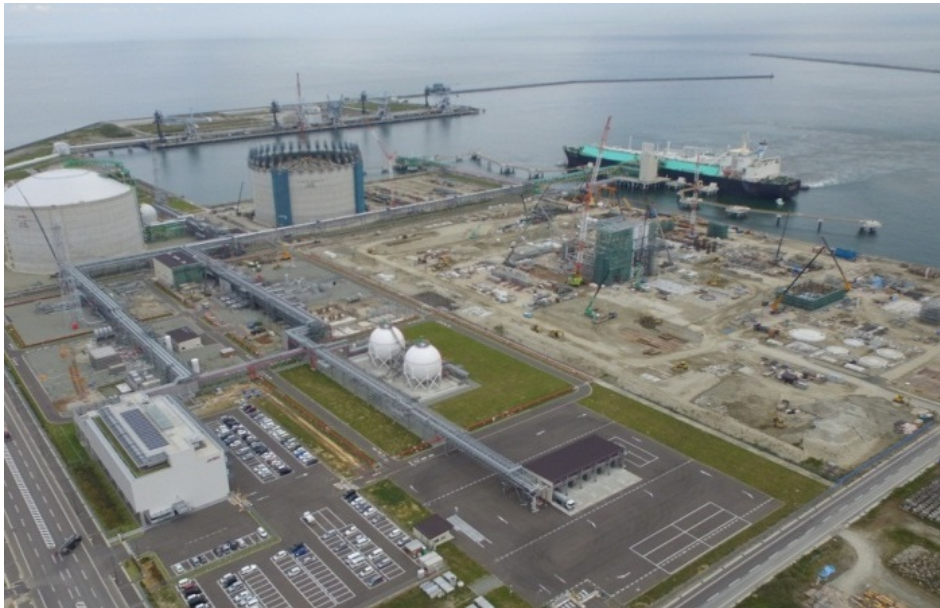
△Soma LNG Terminal and Fukushima Natural Gas Power Plant as of October, 2018
