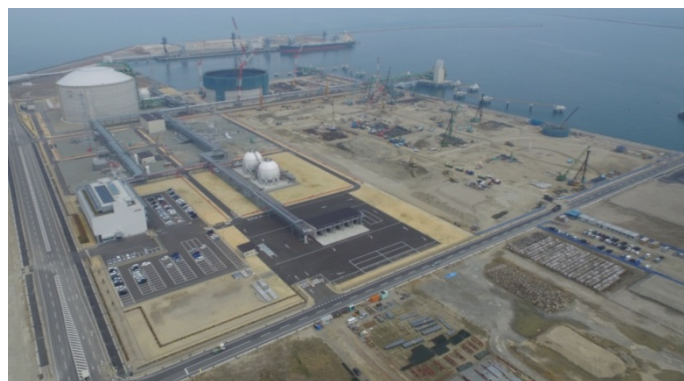
Bird View of Soma LNG Terminal: as of March, 2018
