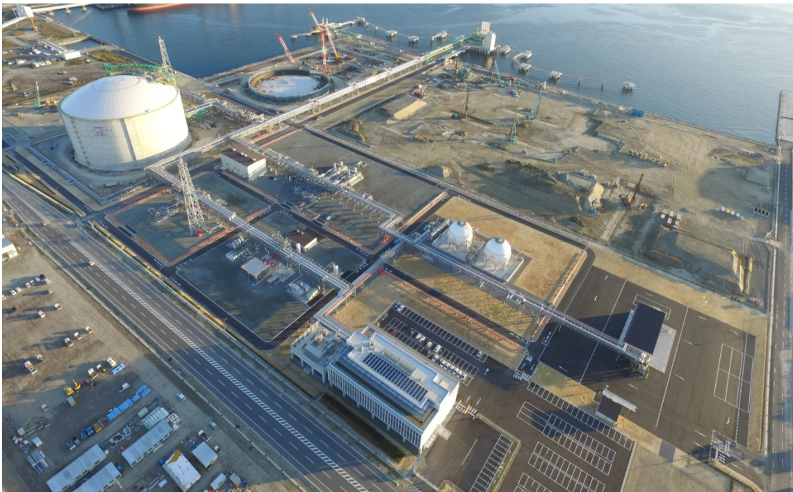
(Bird View of the Soma LNG Terminal: as of November, 2017)
