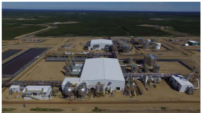
Photo (Right side): Bird-eye View of Central Processing Facility
