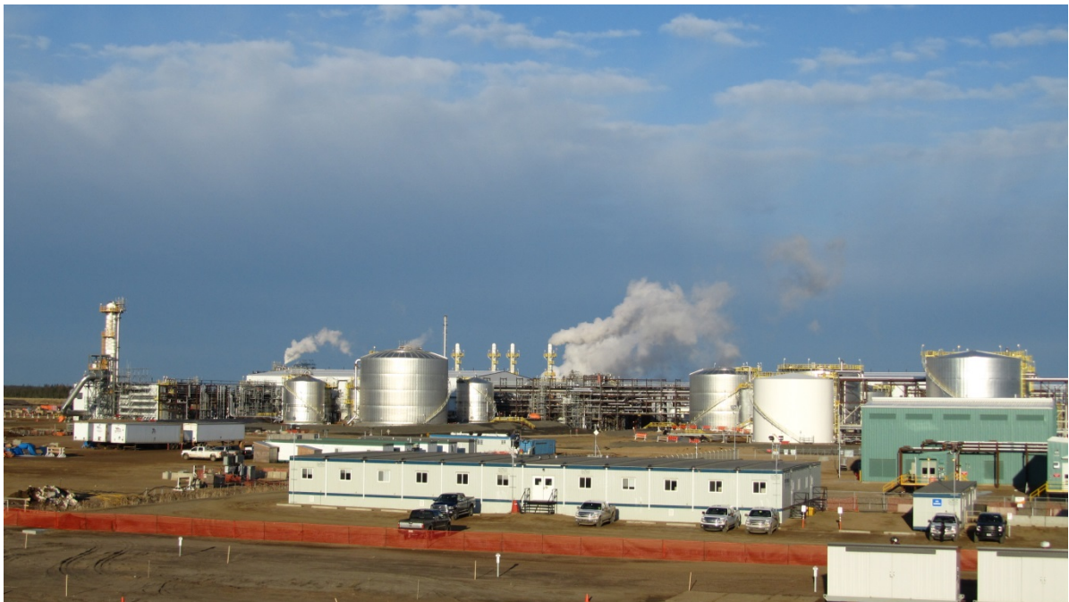
(Picture 1: the Central Processing Facility has started providing steam to the horizontal wells)
