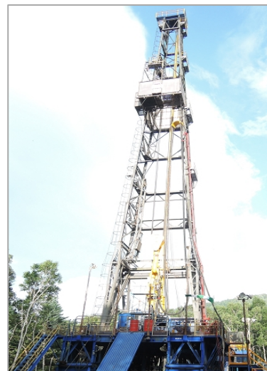
【Drilling Operation of “Musadake SMMG-1D”】
