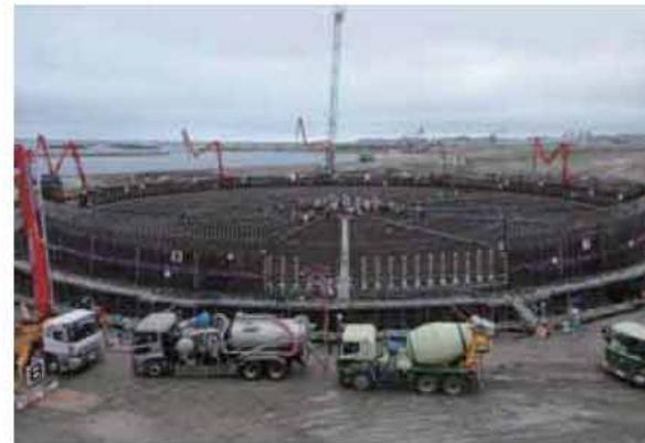
Laying the concrete for the tank's deck slab
