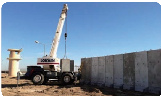
T-wall construction
