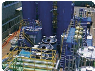
Pit-wastewater processing system
