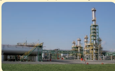
Yufutsu LPG Plant (CO 2 Reduction Facility)
