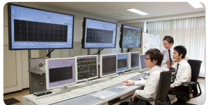
Nagaoka Pipeline Monitoring Center
