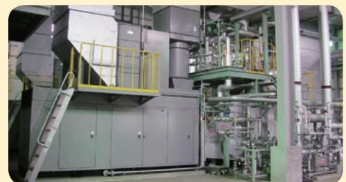
Gas turbine electricity generator at the co-generation system
