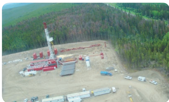
Drilling at a Canadian shale gas project site.
