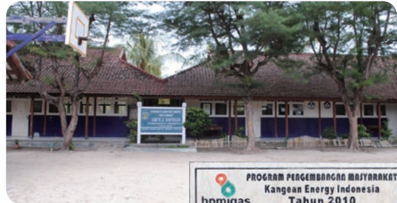
School after repair
