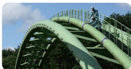
A gas pipeline bridge linking Niigata and Sendai.
