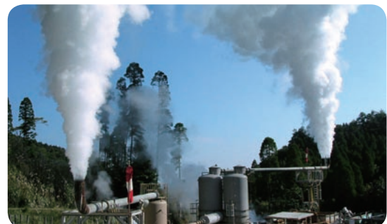
NEDO Geothermal Development Promotion Survey 2001-2004, Kirishima-Eboshidake area geological survey, blowout test undertaken by JAPEX
