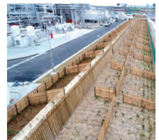
Potted saplings that have been planted in the ground (greening construction)
