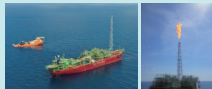
FPU located at Terang gas field in Kangean PSC area
