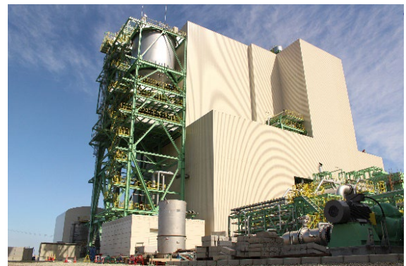
Panoramic view of the Ozu Biomass Power Plant
