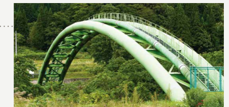
△ Niigata-Sendai Gas Pipeline
