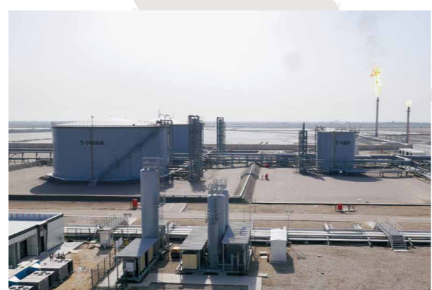
△ Central production facility
